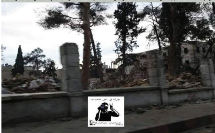
An image showing al-Saraya building in al-Bab city after being targeted, source of image Aleppo, al-Bab Lens page.
