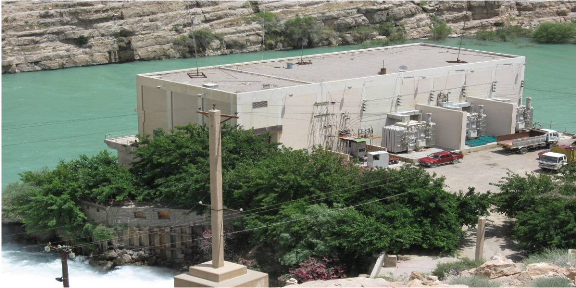
The Kajakai Dam power house in Helmand Province. (Photo by the Office of Inspector General, May 2009.)
