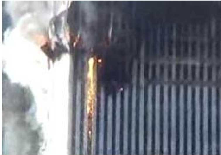
Figure A.1: Molten steel pouring from the burning World Trade Center. An ordinary fire is not hot enough to melt steel.
