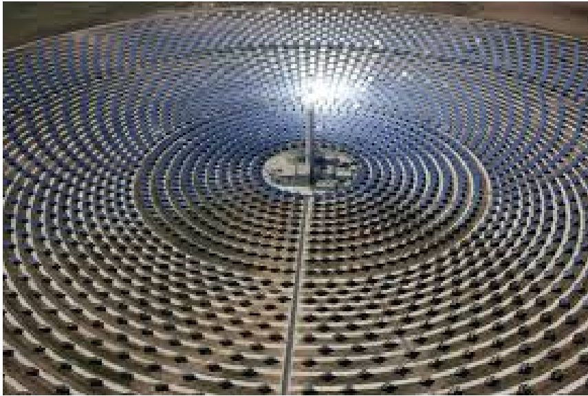
Figure 6.6: A solar thermal power plant. Arrays of heliostatic reflectors concentrate the sun's rays onto molten salt in the tower. The plant produces electricity at night because the salt remains hot.
