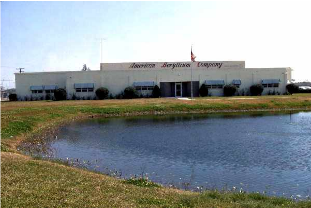
American Beryllium Company at 1600 Tallevast Rd. in Sarasota, Florida, 1969. The American Beryllium Company manufactured ultra-precision machine parts from beryllium-containing metals at 1600 Tallevast Road. Disposal of solvents, including trichloroethylene, resulted in groundwater contamination. In 1996, the Lockheed Martin Corporation purchased American Beryllium and ceased operations. Source: Florida Memory
