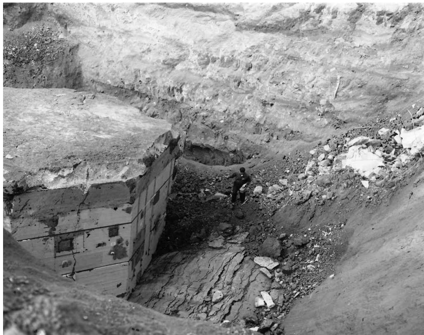
Argonne history: Chicago Pile-3 Demolition November 7, 1955
