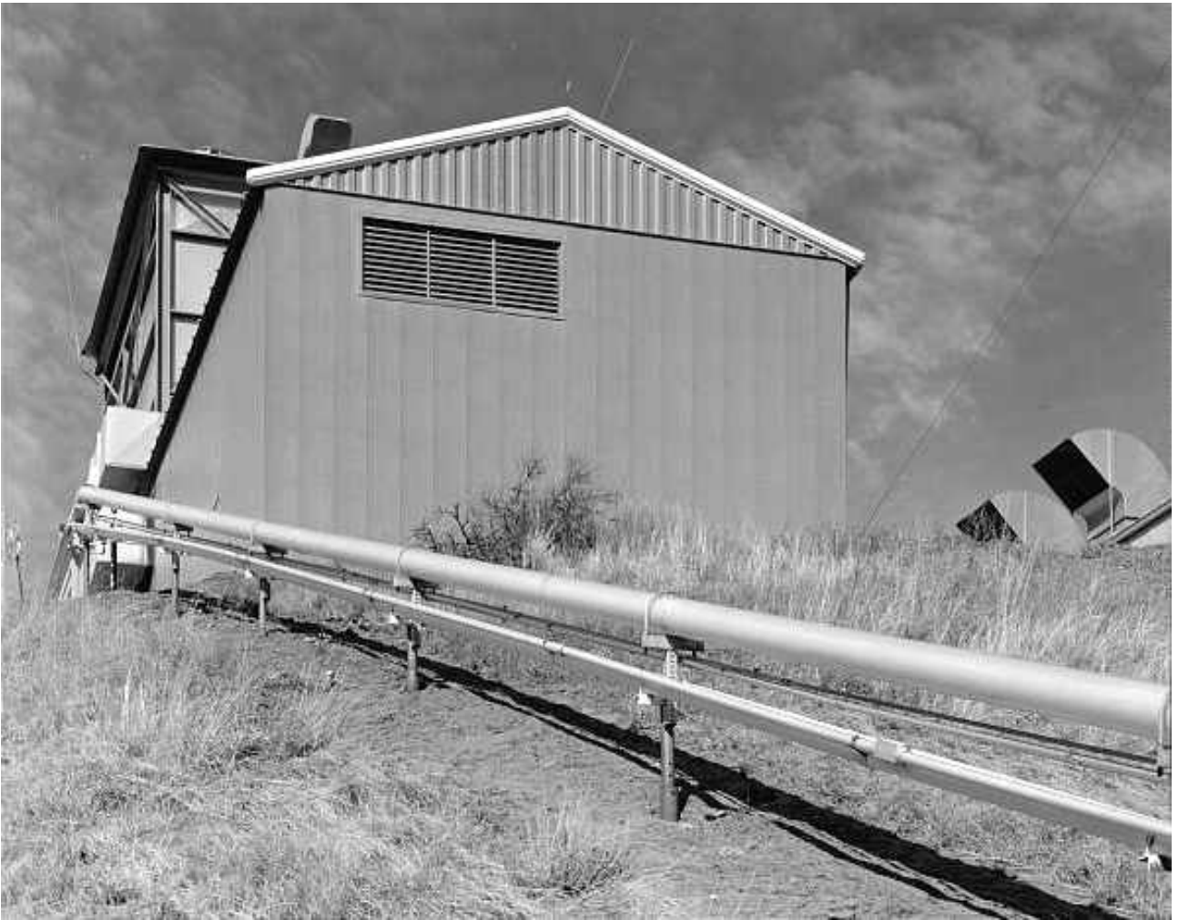
Exterior view of south wall of Oxidizer Conditioning Structure (T-28D), looking north. The taller structure immediately to the rear in the upper left background is the Long-Term Oxidizer Silo (T-28B). Source: Library of Congress.
