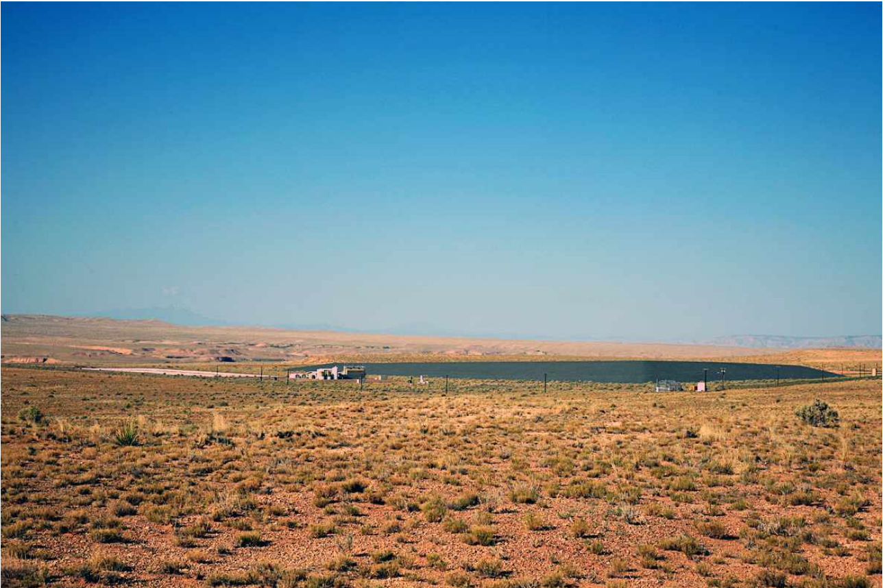
Tailings from a uranium mine and mill, currently undergoing clean-up as part of the Uranium Mill Tailings Remediation Act Project. The site covers approximately 105 acres, and is located on part of the Bennett-Freeze District land, bordering on the Navajo Nation and lands of the Hopi Tribe. The Tuba City mill was built in 1955-56 by Rare Metals Corporation of America and included limited employee housing at the site. The Rare Metals Corporation merged with the El Paso Natural Gas Company in 1962 and operated the mill
