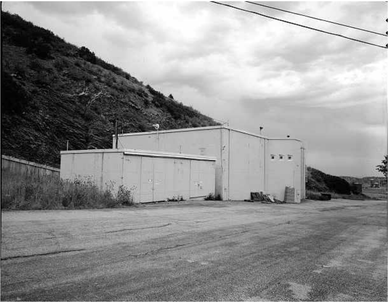
•CO Glenn L. Martin Company, Titan Missile Test Facilities Lakewood vicinity, Jefferson AWE including Glenn L. Martin Company, Titan Missile Test Facilities, CaptiveTest Stand D-3 and Glenn L. Martin Company, Titan Missile Test Facilities, Captive Test Stand D-4
