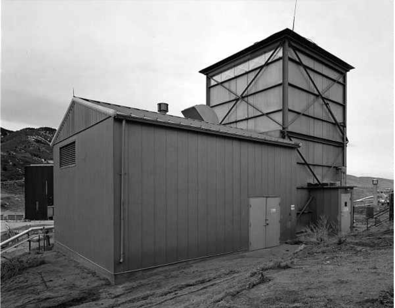
Exterior view of south and east walls of Oxidizer Conditioning Structure (T-28D), looking northwest. This structure was designed to condition nitrogen tetroxide, the oxidizer used in the Titan II's fuel system, to specified temperatures. The taller structure to the rear is the Long-Term Oxidizer Silo (T-28B).
