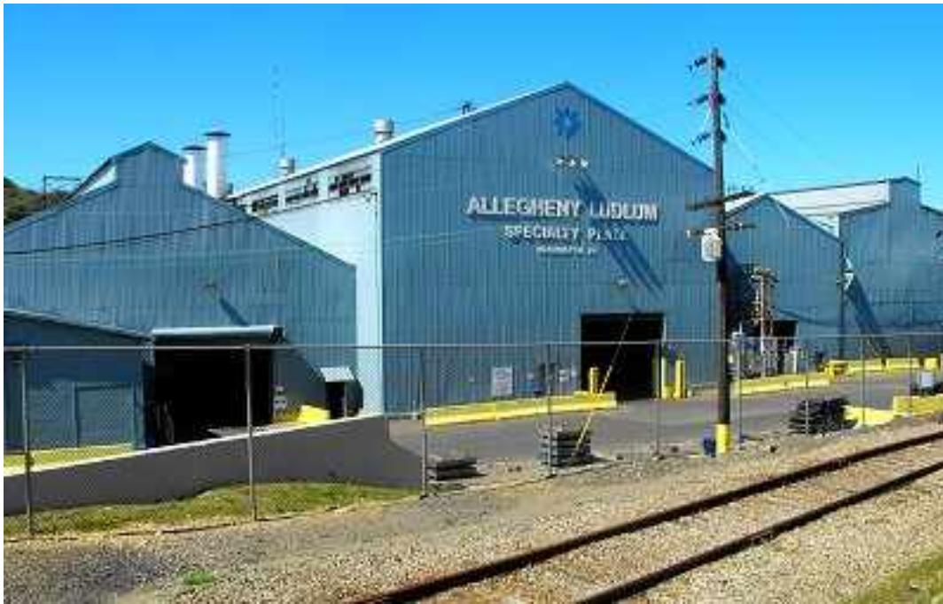
This steel mill in Washington, PA was once Jessop Steel, but was purchased by Allegheny Ludlum in the 1990s.
