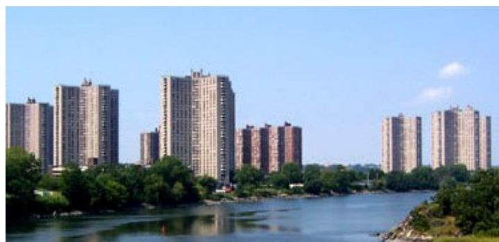
Figure 5.8: Co-op City in The Bronx, New York City is the largest cooperative housing development in the world, with 55,000 people.
