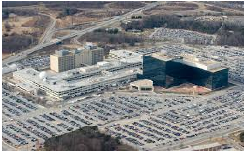
Figure 12.14: These huge buildings in Fort Meade, Maryland, are the main headquarters of NSA.
