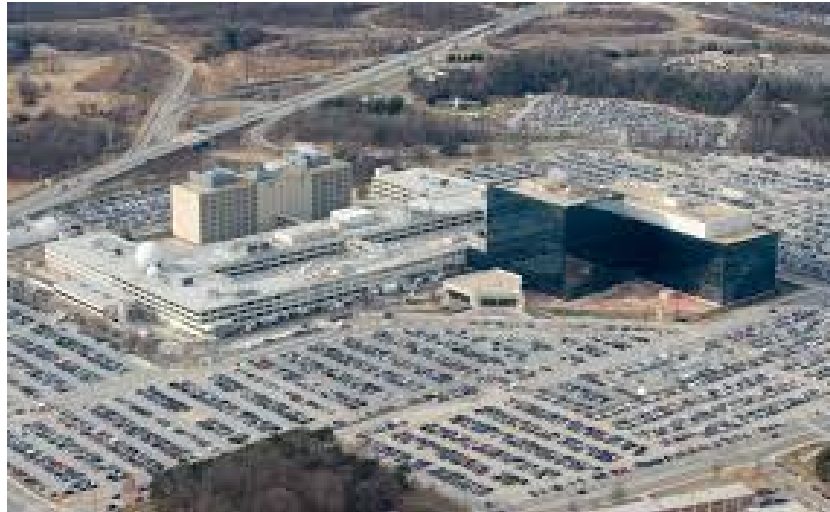
Figure 8.6: These huge buildings in Fort Meade, Maryland, are the main headquarters of NSA.
