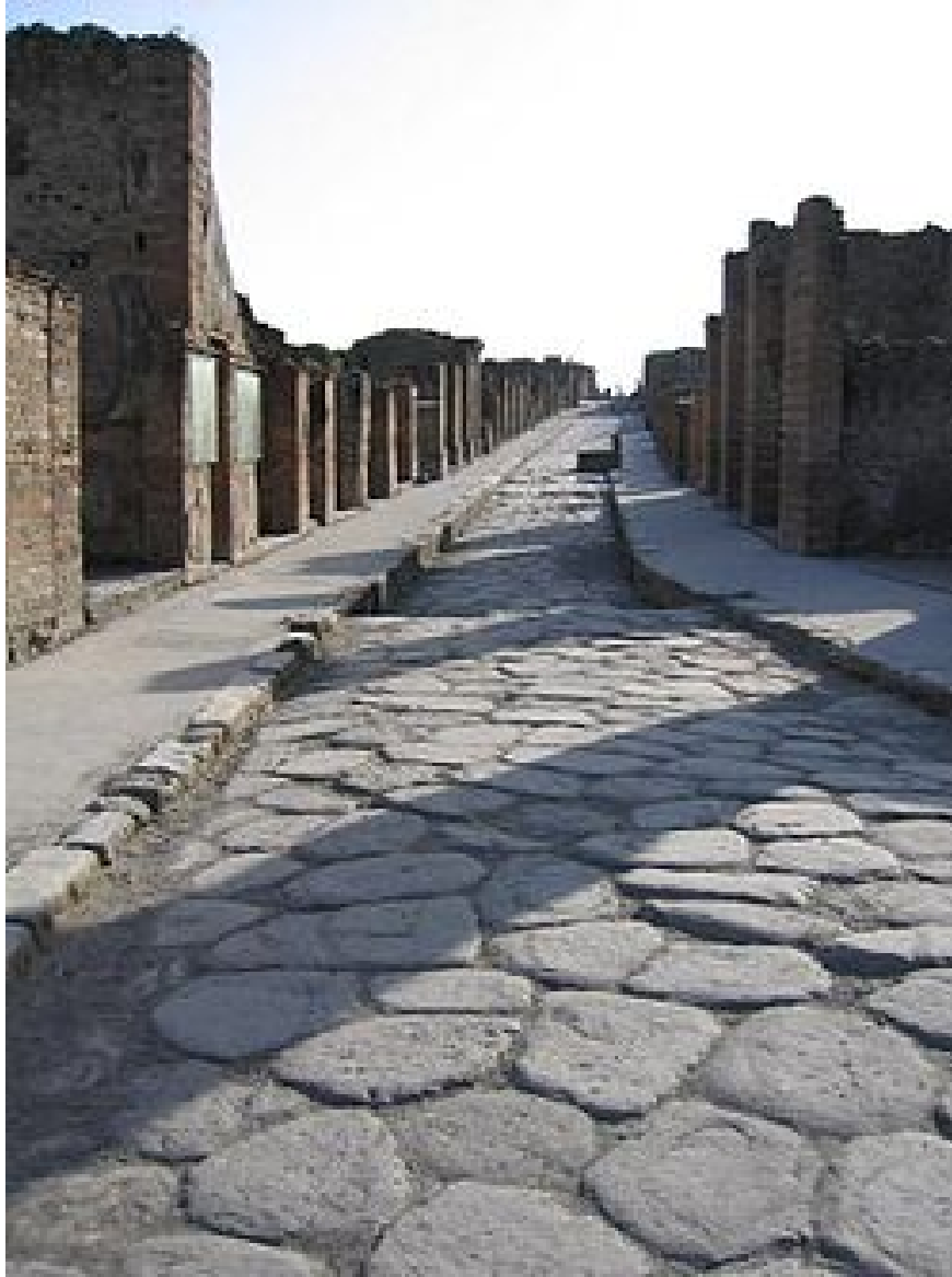
Figure 2.14: A Roman street in Pompeii. At the peak of Rome's development, the late Empire's 113 provinces were interconnected by 372 great roads. The total length of these roads was more than 400,000 kilometers (250,000 miles).
