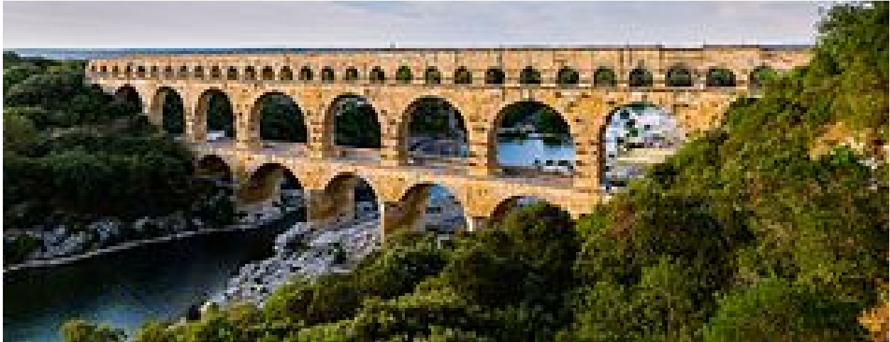
Figure 2.12: A Roman aqueduct: The multiple arches of the Pont du Gard in Roman Gaul (modern-day southern France). The upper tier encloses an aqueduct that carried water to Nimes in Roman times; its lower tier was expanded in the 1740s to carry a wide road across the river.
