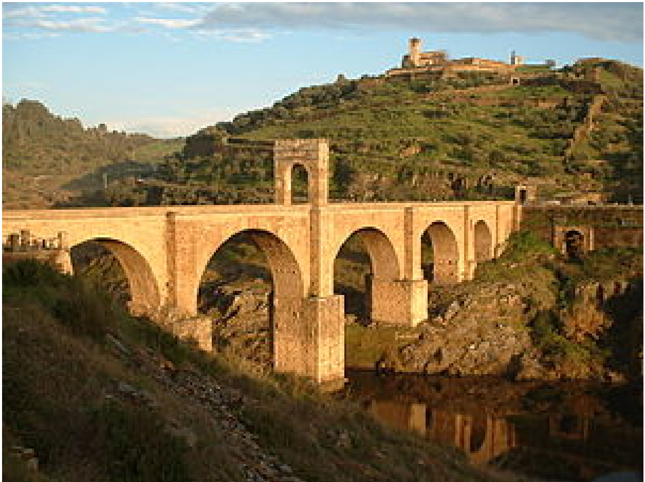
Figure 2.11: The Alcántara Bridge, Spain, a masterpiece of ancient bridge building.
