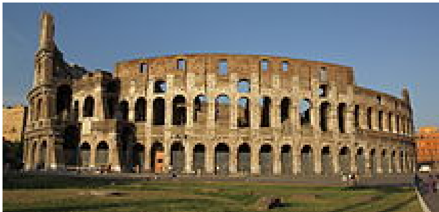
Figure 2.13: The exterior of the Colosseum, showing the partially intact outer wall (left) and the mostly intact inner wall (center and right). The outer wall is estimated to have required over 100,000 cubic meters (3,531,467 cubic feet) of travertine stone which were set without mortar; they were held together by 300 tons of iron clamps.
