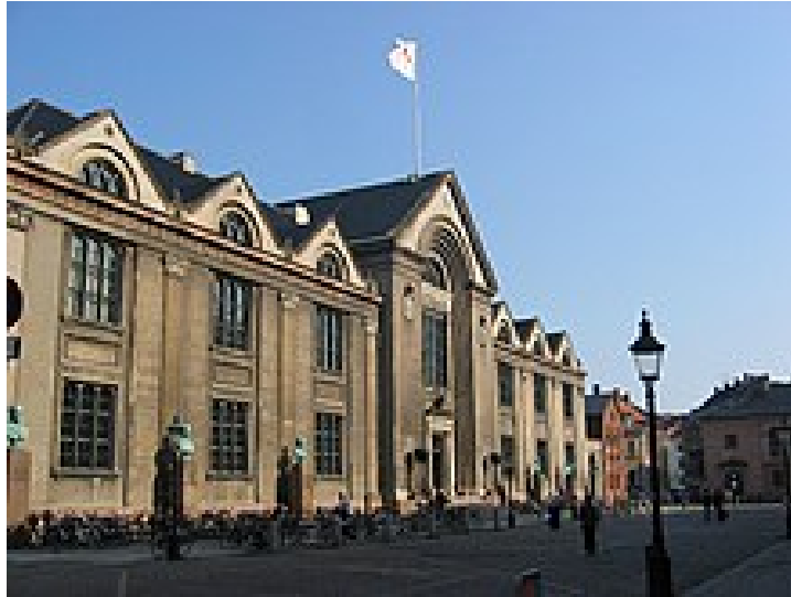
Figure 6.25: University of Copenhagen buildings at Frue Plads.
