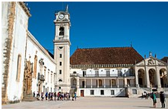
Figure 6.9: Some of the University buildings.
