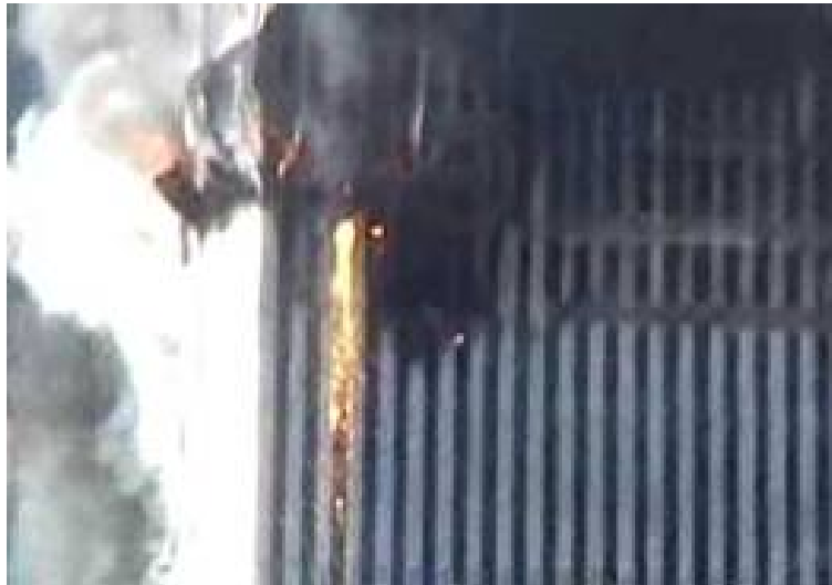
Figure 7.4: Molten steel pouring from one of the twin towers before its collapse.
