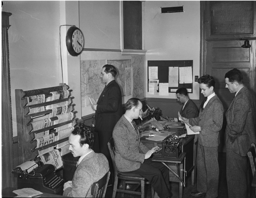
Figure 6.15: Journalists at work in Montreal in the 1940s. Today, the mass media form an extremely important part of our total educational system. (Public domain)
