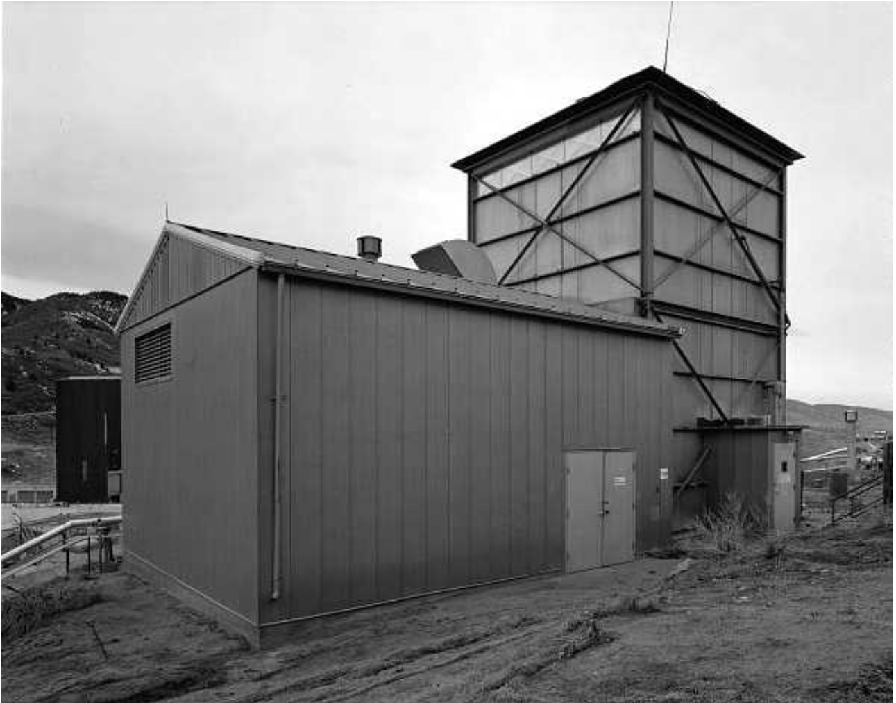
Exterior view of south and east walls of Oxidizer Conditioning Structure (T-28D), looking northwest. This structure was designed to condition nitrogen tetroxide, the oxidizer used in the Titan II's fuel system, to specified temperatures. The taller structure to the rear is the Long-Term Oxidizer Silo (T-28B). Source: Library of Congress.
