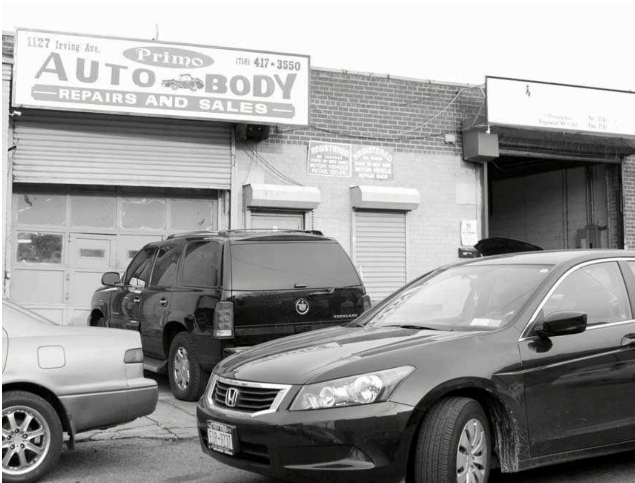
This auto body shop located at 1127 Irving Ave. on the Brooklyn/Queens border in Ridgewood was once the site of the Wolff-Alport Chemical Corporation. The New York City Department of Health is currently investigating radioactive contamination at and in the immediate vicinity of the site, where Wolff-Alport processed materials during the 1940s and 1950s that produced radioactive byproducts.
