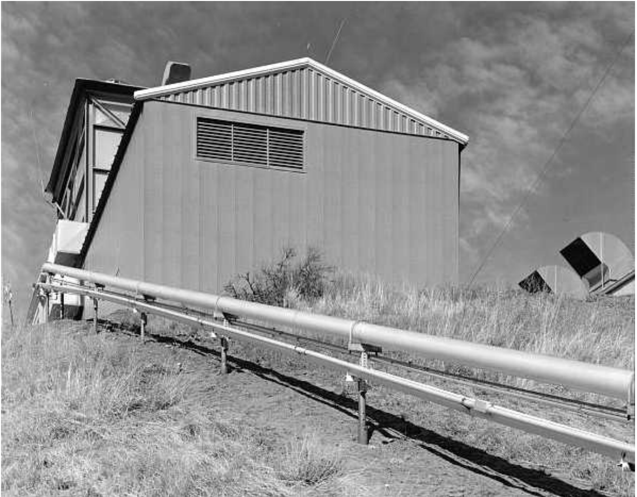
Exterior view of south wall of Oxidizer Conditioning Structure (T-28D), looking north. The taller structure immediately to the rear in the upper left background is the Long-Term Oxidizer Silo (T-28B). Source: Library of Congress.
