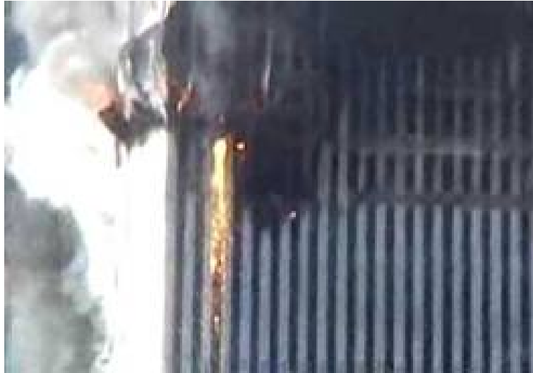
Figure 9.4: Molten steel pouring from one of the twin towers before its collapse.
